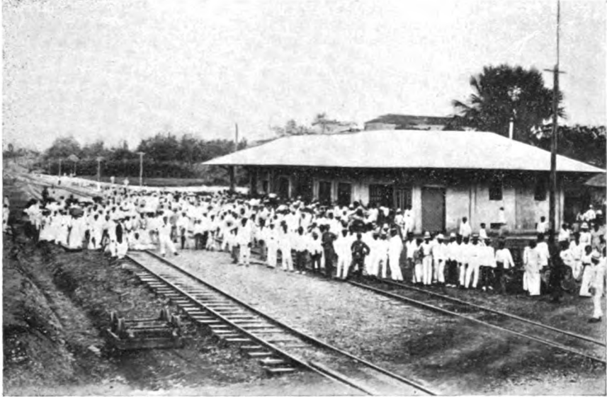
STATION ON A NEWLY CONSTRUCTED RAILROAD IN THE PHILIPPINES
